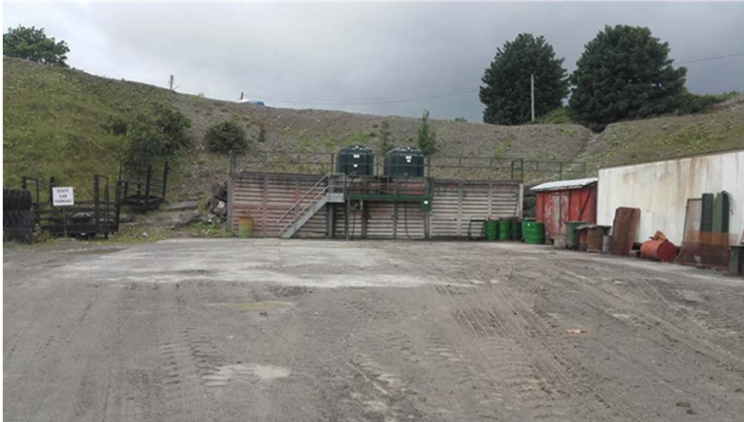
Figure 8-4: Above Ground Fuel storage and Refuelling Area
