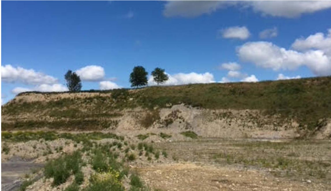
Plate 13.7: Restored Side Slopes North Eastern Boundary
