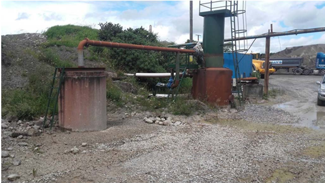
Figure 8-3: Photograph of washing plant wells / sumps
